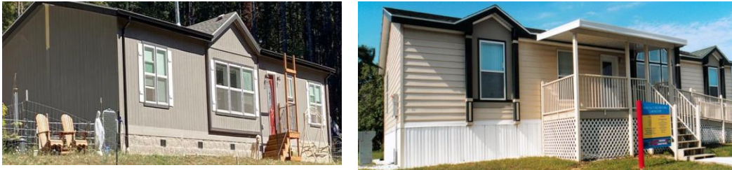
Figure 1. Pictures of MH located in Oregon (left) and Central Florida (right).
